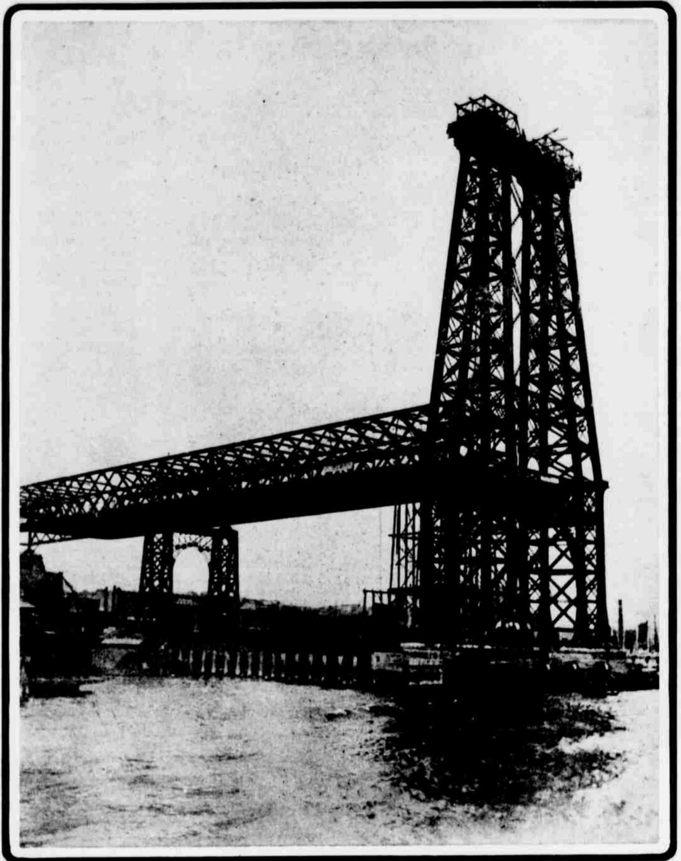
MANHATTAN END OF NEW EAST RIVER BRIDGE, LOOKING FROM THE RIVER.
