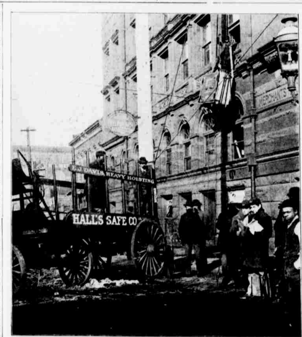
Safe being hoisted by E. J. Davis for J. J. Deright, agent for Hall's Safes, in Merchant's National Bank Building, for Omaha Street Railway Company.
