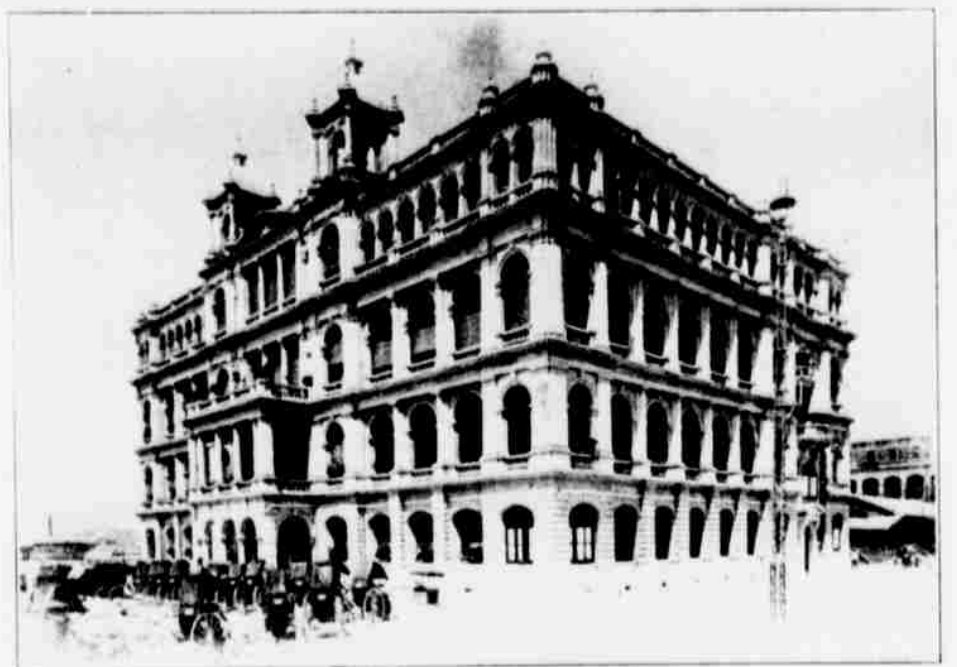
VICTORIA A CITY OF CLUBS—BUILDING OF HONG KONG CLUB—IT COST $350,000.
