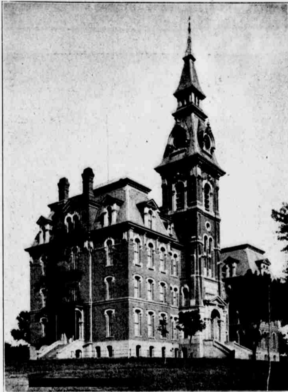
OMAHA HIGH SCHOOL BUILDING—TO BE REPLACED BY NEW BUILDING IN COURSE OF CONSTRUCTION.
