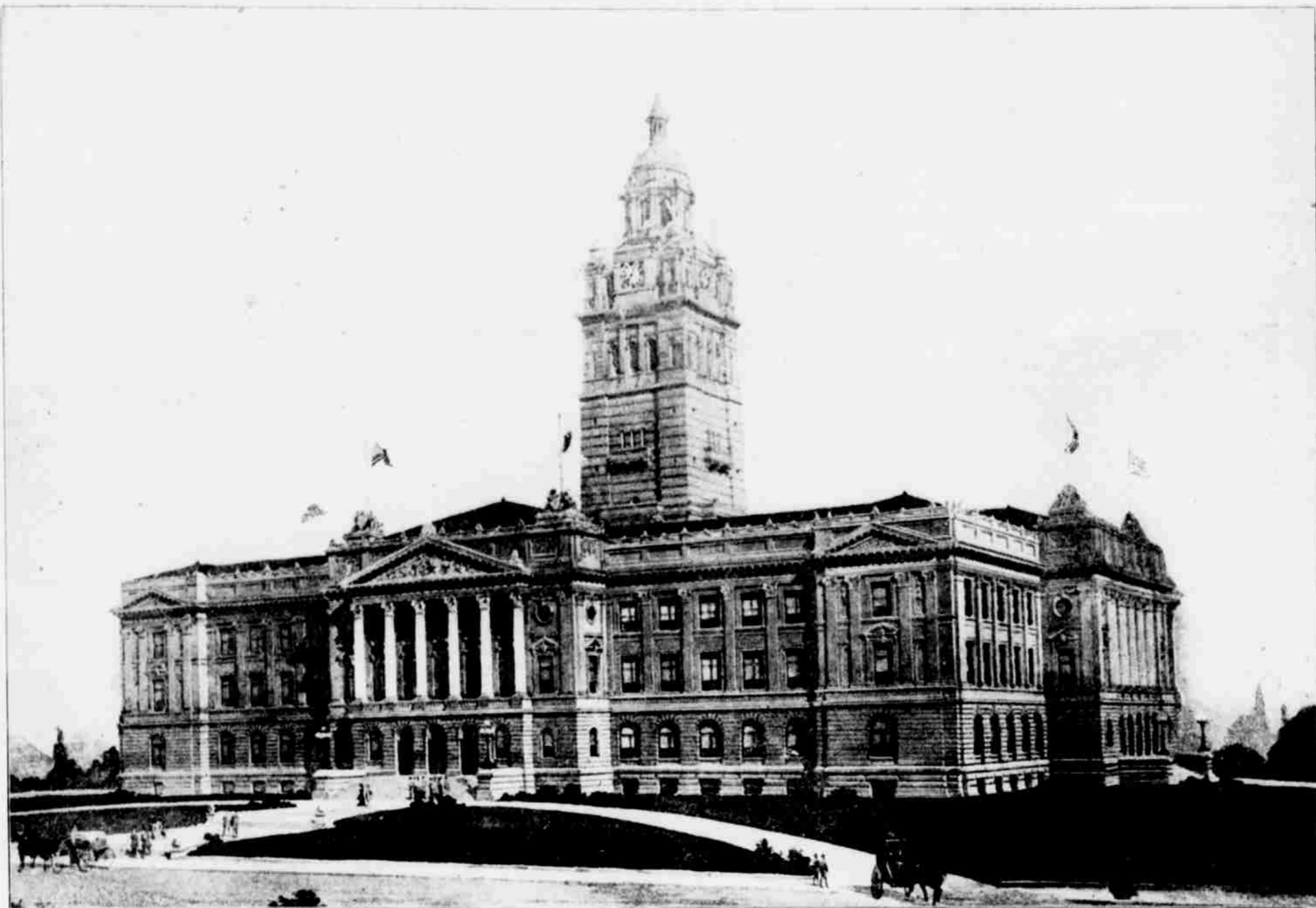
OMAHA HIGH SCHOOL WHEN COMPLETED.
