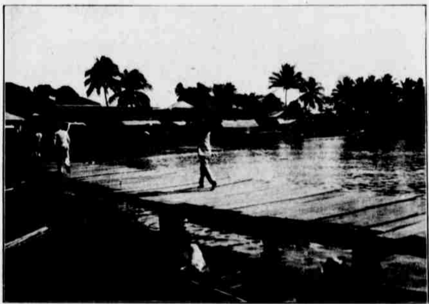
ROSEWOOD BRIDGE AT ZAMBOANGA.
