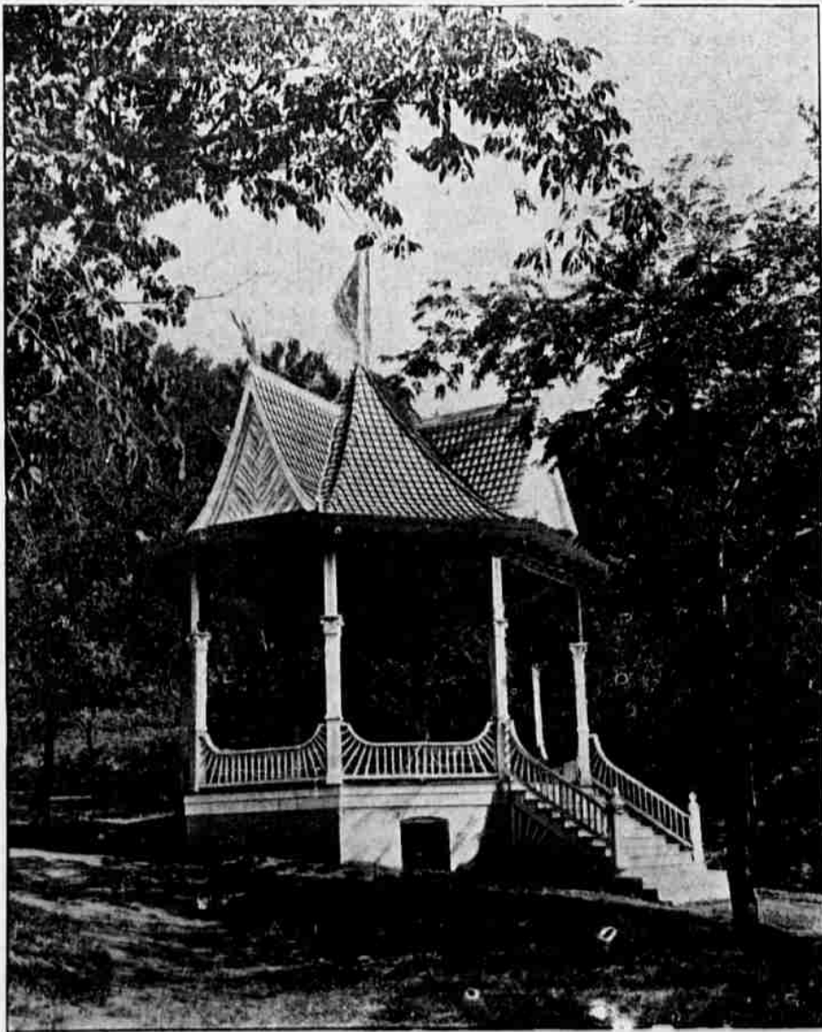
BAND STAND, FAIRMOUNT PARK, COUNCIL BLUFFS—J. C. AND W. WOODWARD, ARCHITECTS.
