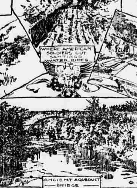
SANTIAGO'S WATER WORKS.
