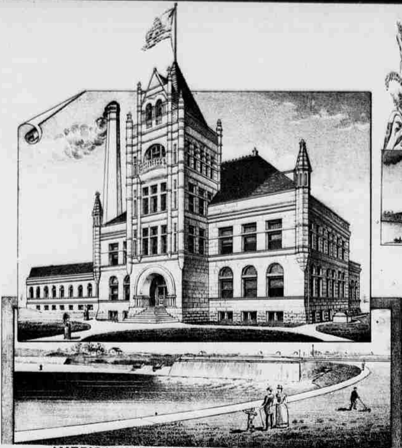
AMERICAN WATER WORKS PUMPING STATION.
