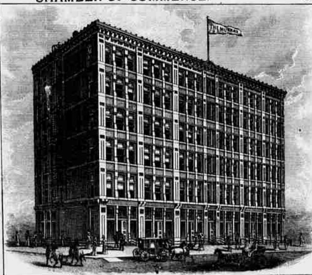
MURRAY HOTEL. ERECTED 1889.
