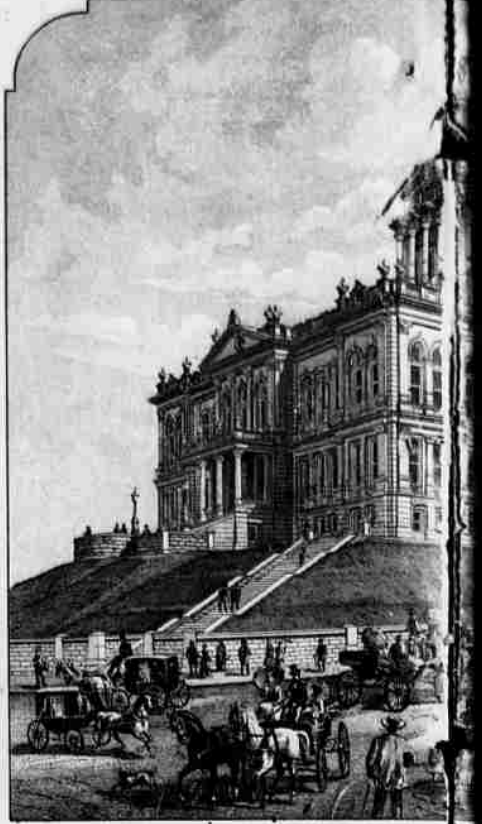
DOUGLAS COUNTY COURTHOUSE.
