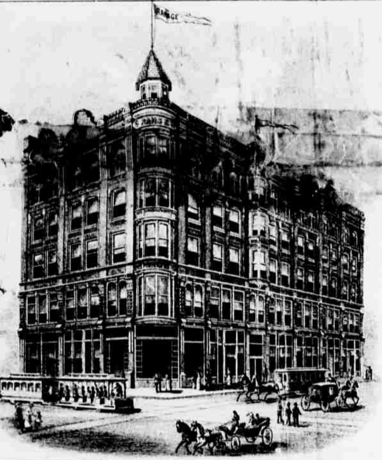
FRANK RANGES BUILDING. ERECTED 1887.
