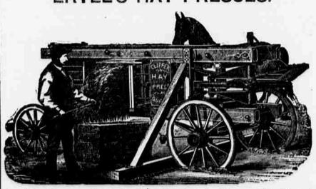
With no Hay Presses of any kind can the amount of work produced, such little expense, (ten tons of hay and over to load ra'hoad box car,) as can be done with the Ertel Improved Machines. Warranted or no sale. For illuistrated new circular address, a 11em ERTEL & CO., Quincy, illinois.
