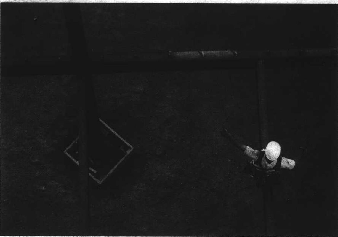
A WORKER from Sampson General Contractors Inc. balances on a beam Thursday afternoon at the construction site of a new parking garage. The garage, at 12th and Q streets, will have a university art gallery inside. LIZ MEACHAM/DN
