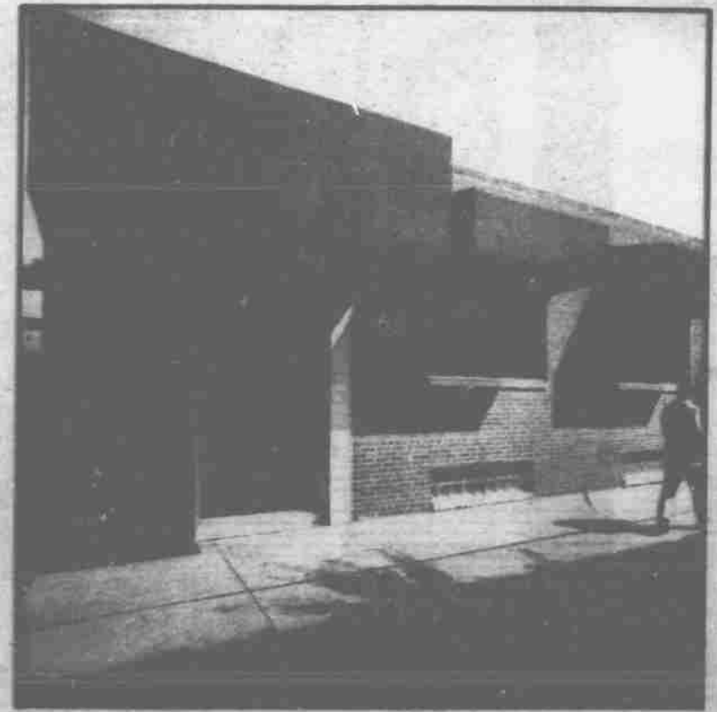
1630 Q St. building
