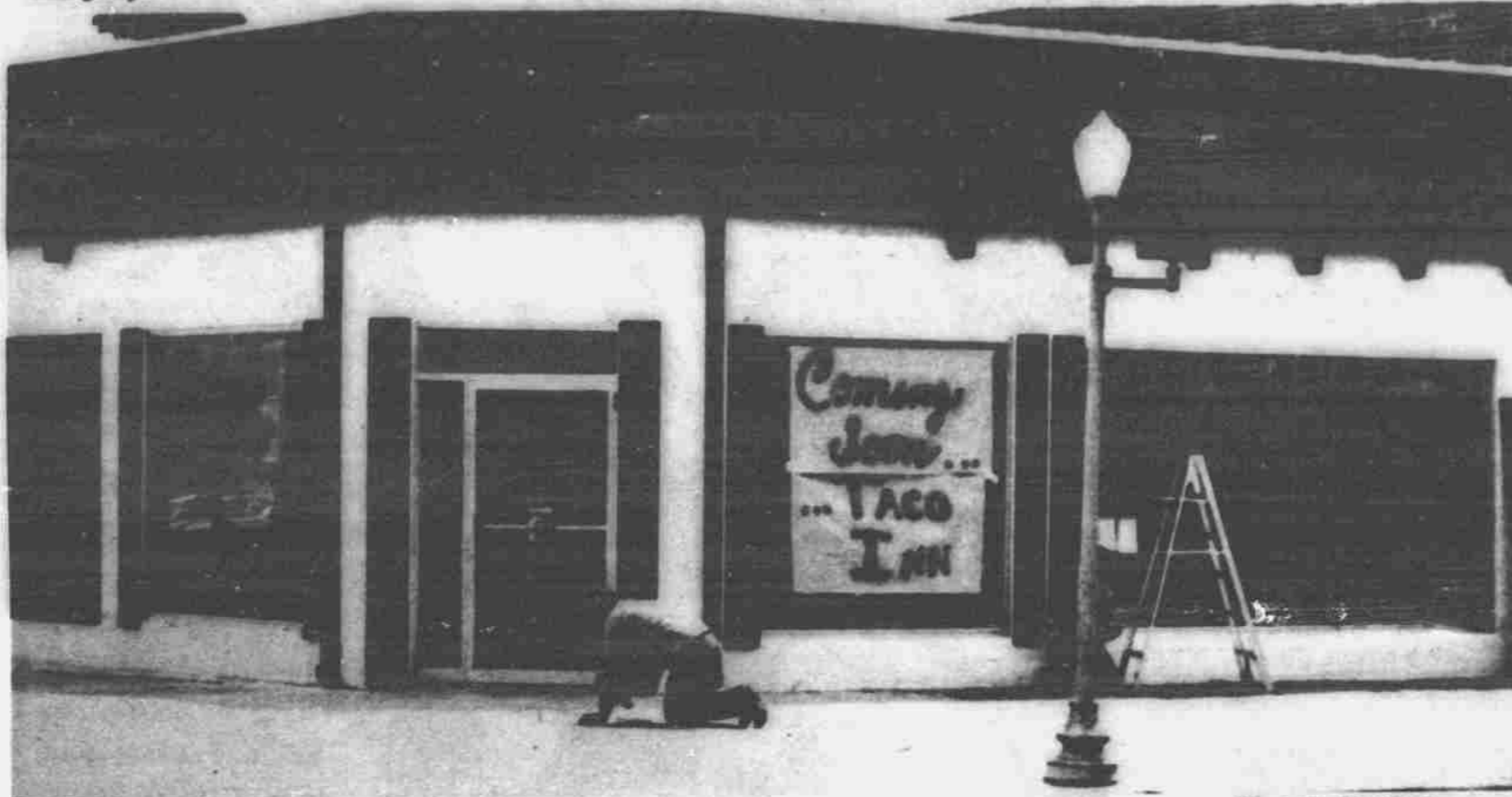
A worker puts the finishing touches on the Taco Inn, 1245 R St., opening Aug. 1.
