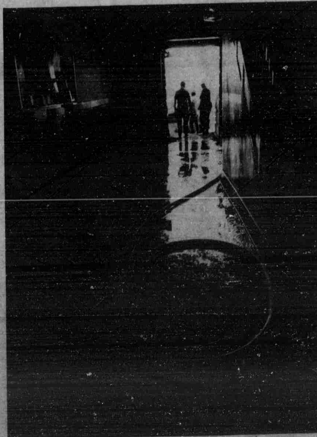
The efforts of firemen to extinguish the fire in the East Campus Plant Industry Bldg. caused water damage on the building's first floor.
