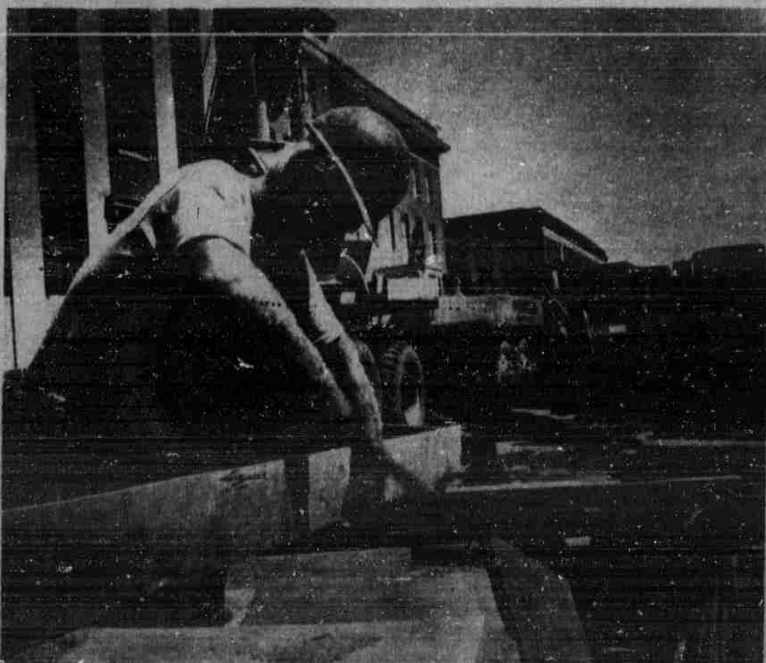
Construction workers battle the blistering summer heat during work on the new Life Sciences Bldg. west of Hamilton Hall.
