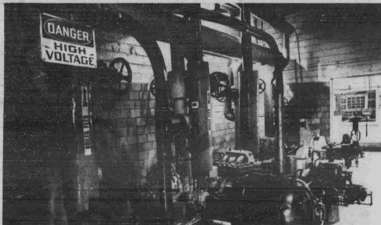
UNL power plant
