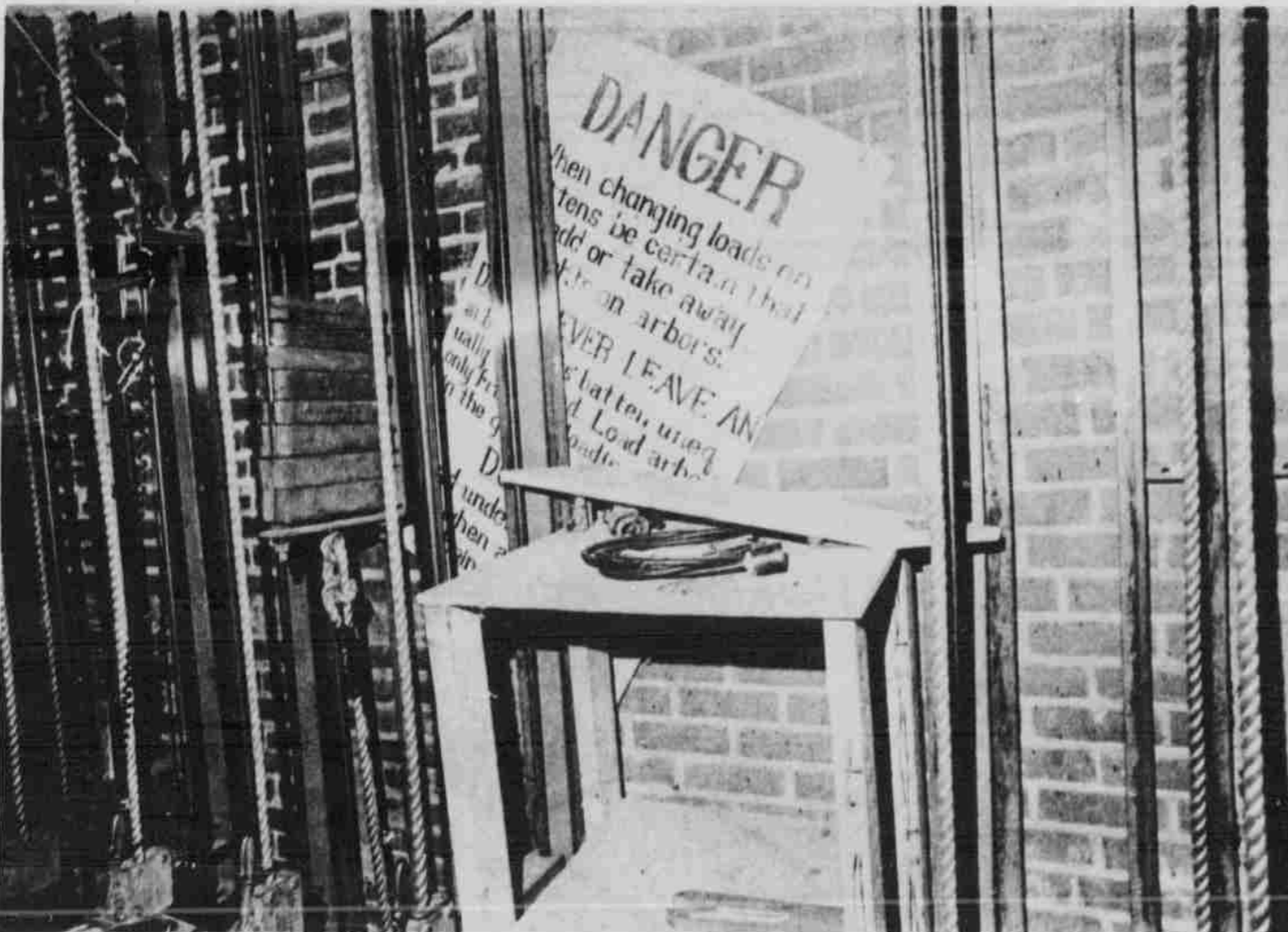
Temple . . . "From a fire safety standpoint this building is in a very poor condition."
