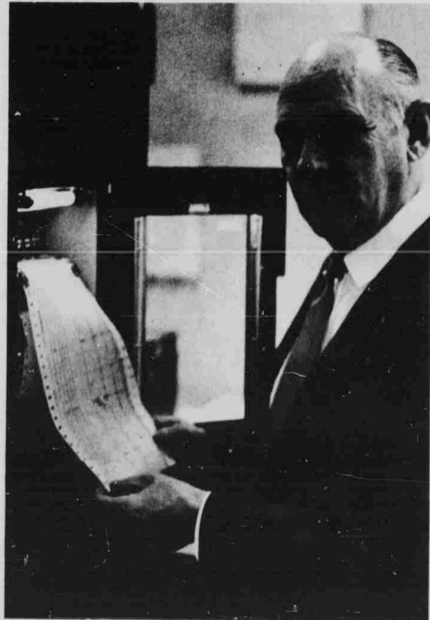
Climatologist Richard E. Myers takes a reading from the weather event recorder. The machine measures wind direction and speed, amount of precipitation, amount of sunlight per day, temperature and barometric pressure.
