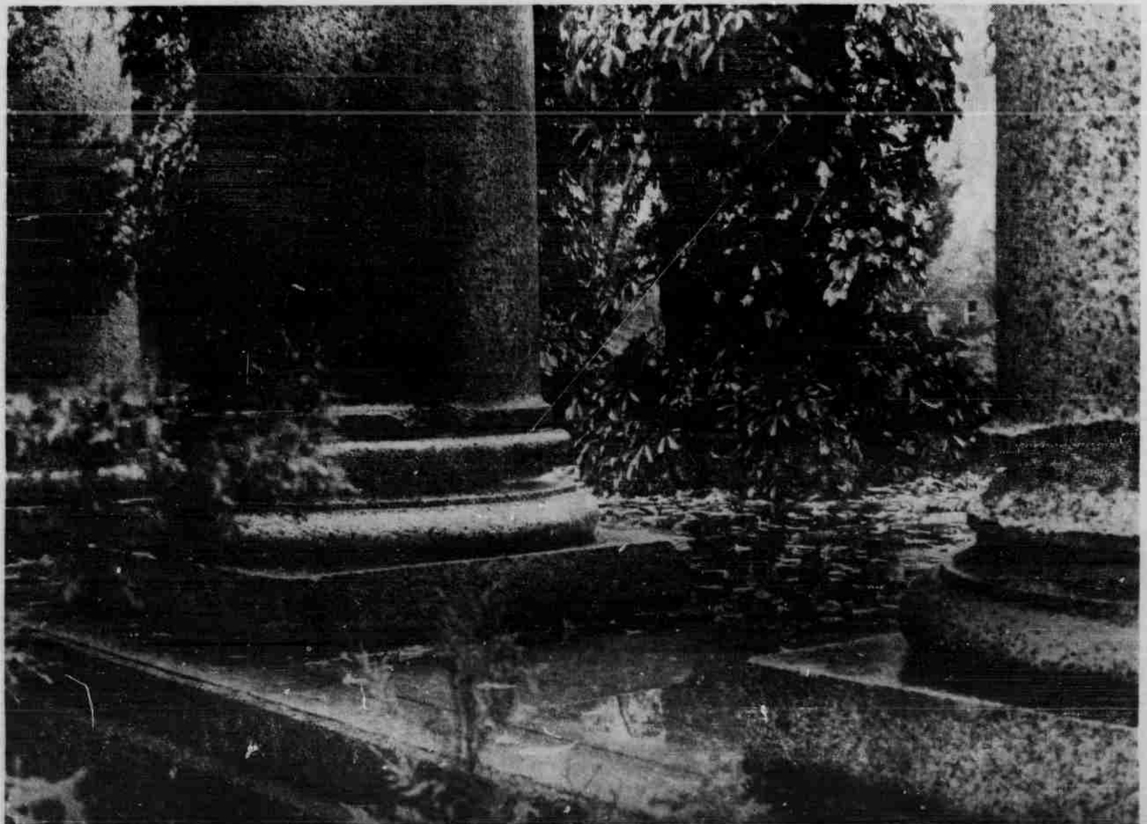
... Fall to Form a rusty flooring for the Column's.
