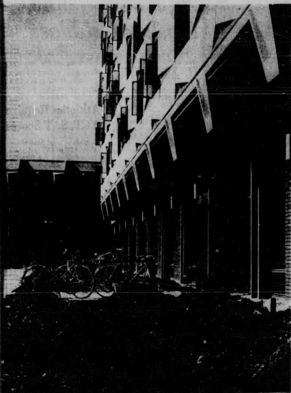
HARPER PRESENTS VIVID CONTRASTS . . . as final touches bring its completion close to reality. Photo by Mike Hayman
