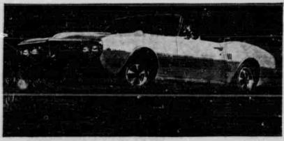
Firebird HO. HO stands for High Output. As a split second behind the wheel will attest to. The Firebird HO boasts a 285-hp V-8 with a four-barrel carburetor, dual exhausts and sport striping. Standard stick is a columnmounted three-speed. Naturally, all Firebird options such as Rally wheels and gauge cluster are available.
