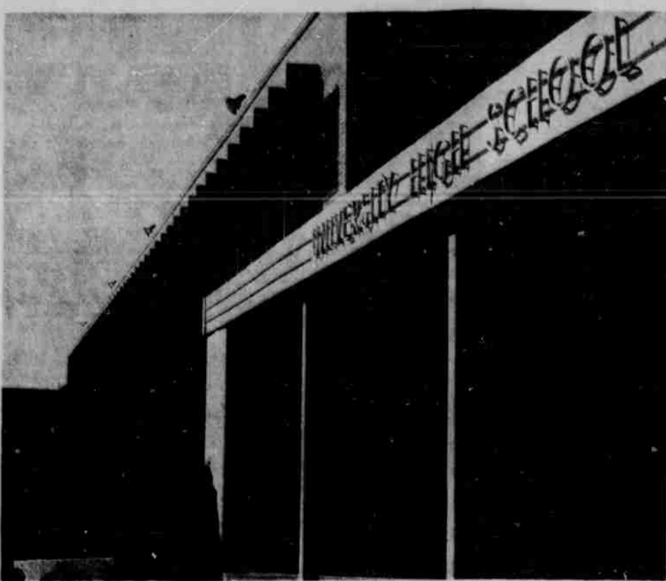
UNIVERSITY HIGH . . . will be renovated after the 1967 summer school session for use by departments of Teacher's College.
