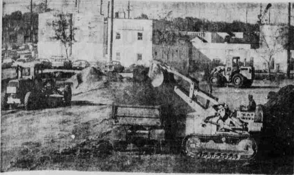
EXCAVATION . . . has begun on the women's physical education field.
