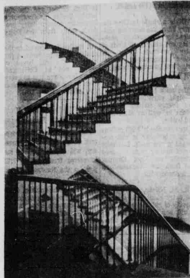
LIKE . . . The scales of justice these stairs fit well in the Social Science building.
