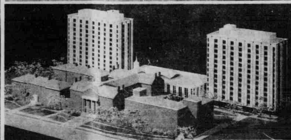
SOON TO BE COMPLETED—The University's new Pound and Cather dormitories.
