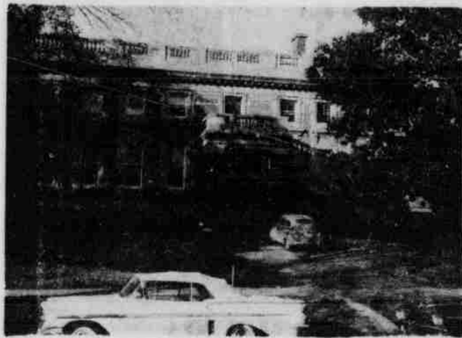
OLD ADMINISTRATION BUILDING . . . In sixty days it will be no more.
