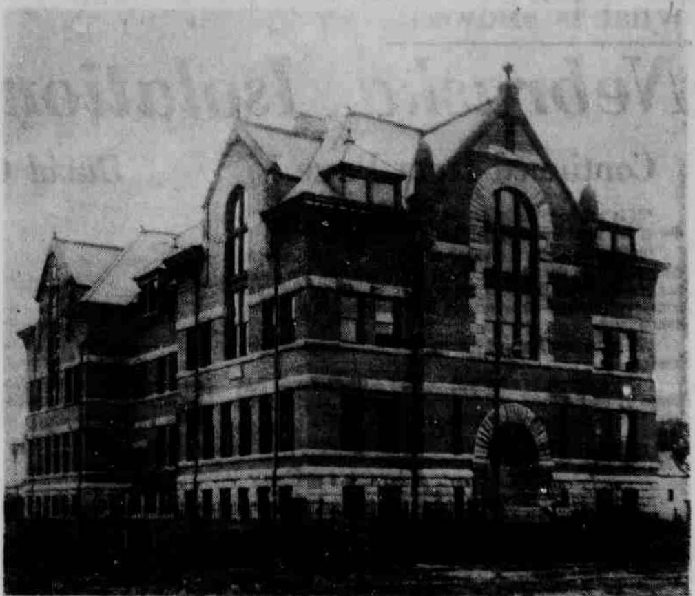
OFF WITH THE OLD—Nebraska Hall, the third building built on the University campus, is shown here shortly after its completion 73 years ago. The building, which once housed the College of Industrial Arts, is now being razed to permit future University construction. The ingredients of its cornerstone, laid in 1888, were uncovered last week.
