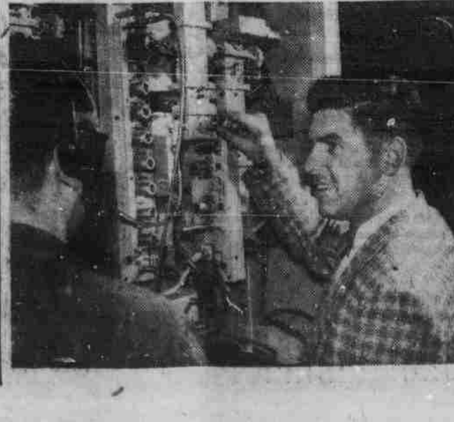
Dick stops by the East Central Office building in Seattle to look at some microwave terminating equipment. It's involved in a 4000 megacycle radio relay system between Seattle and Portland, Oregon.
