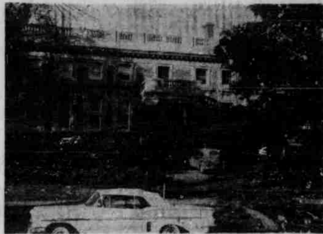
ART BUILDING—The old Administration building will soon be torn down to make room for a new art building.
