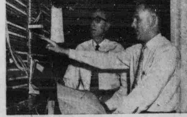
"3:00 p.m. At our toll center we'll soon be adding another test desk to increase our facilities for 'trouble shooting' Long Distance circuits. Here, with our Chief Testboardman, I go over some of the board changes which will have to be made."
