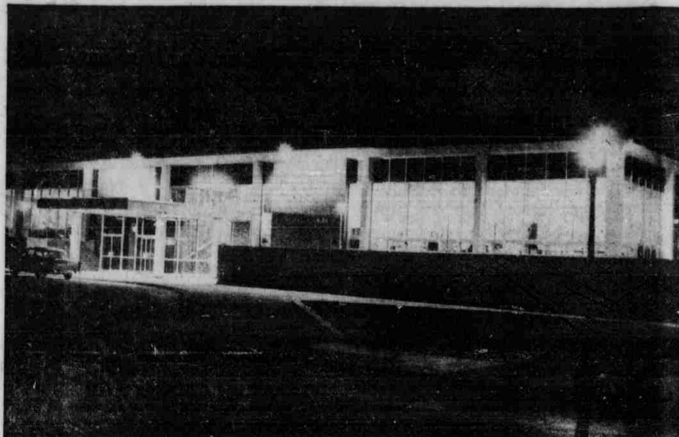
UNION AT NIGHT—Glowing lights set off the modern construction of the new Student Union addition. The $1.3 million structure began to rise in the spring of 1958, after a blanket bond issue including the addition was passed in 1955. Surrounding the brick-faced, plate glass window building is a patio, which will be used for outdoor dancing and other activities.
