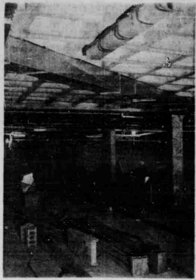
In go the fixtures . . .
