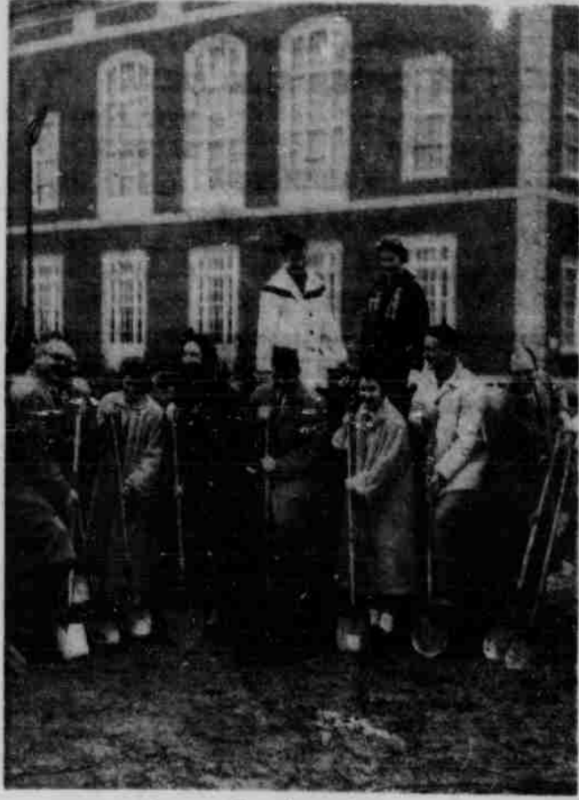
In go the shovels . . .
