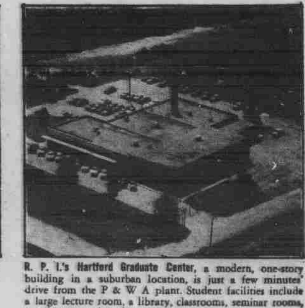
R. P. I.'s Hartford Graduate Center, a modern, one-story building in a suburban location, is just a few minutes drive from the P & W A plant. Student facilities include a large lecture room, a library, classrooms, seminar rooms, a cafeteria, and parking areas.
