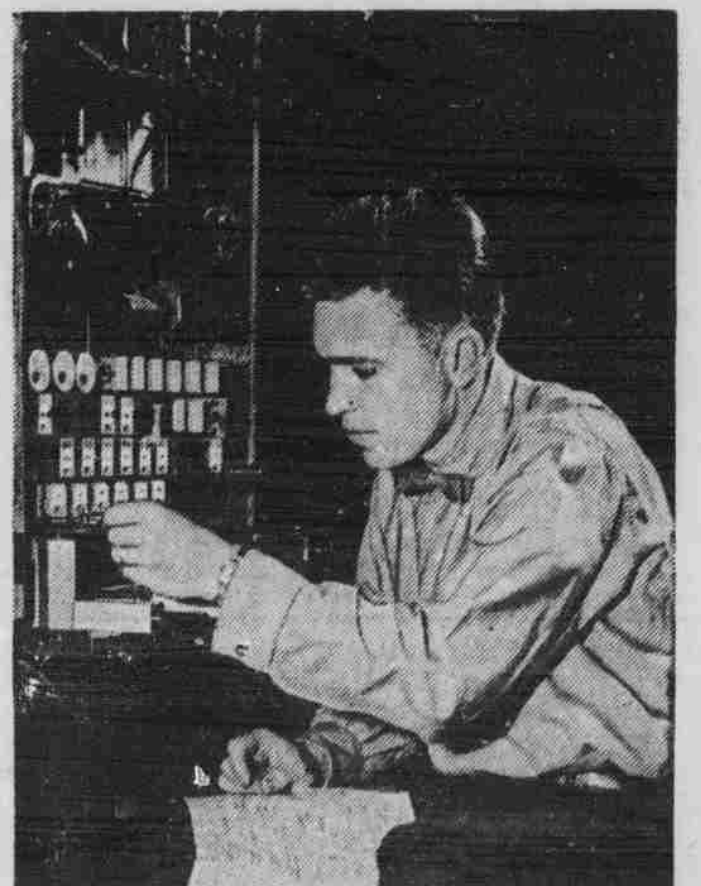
Here Don Garland makes noise distribution measurements with a Level Distribution Recorder
