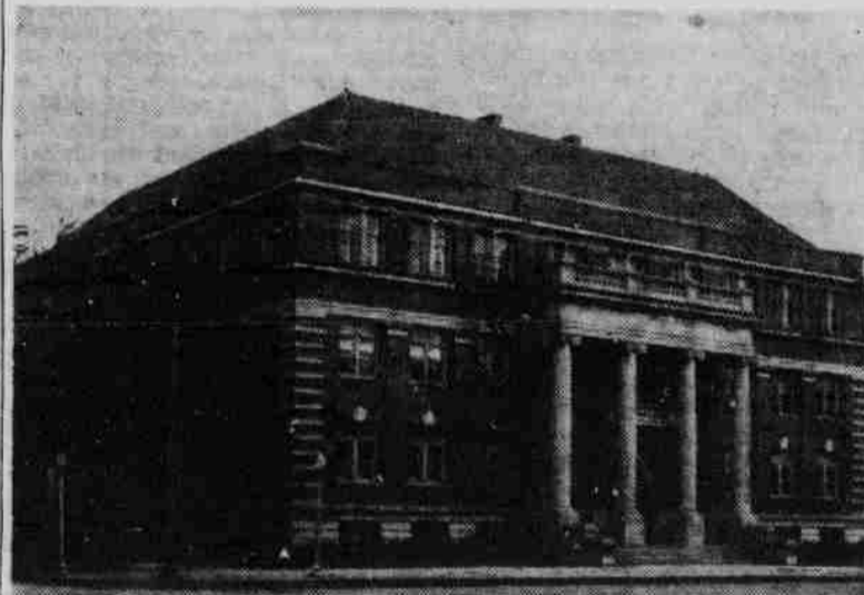
TEMPLE BUILDING . . . The south wing will go under reconstruction. Courtesy Lincoln Star
