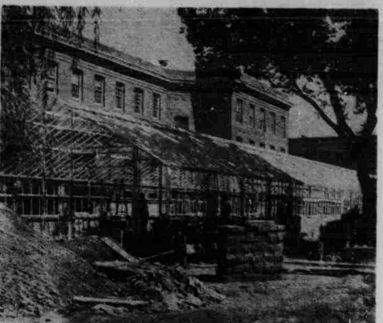
BOTANY GREENHOUSE—Latest construction on city campus, the building will have facilities to study four different botanical functions. The center portion will be built of heat resistant glass. Heat will be controlled by an automatic heating system consisting of steam heat from the walls, suspended blower units and ventilators in the roof.
