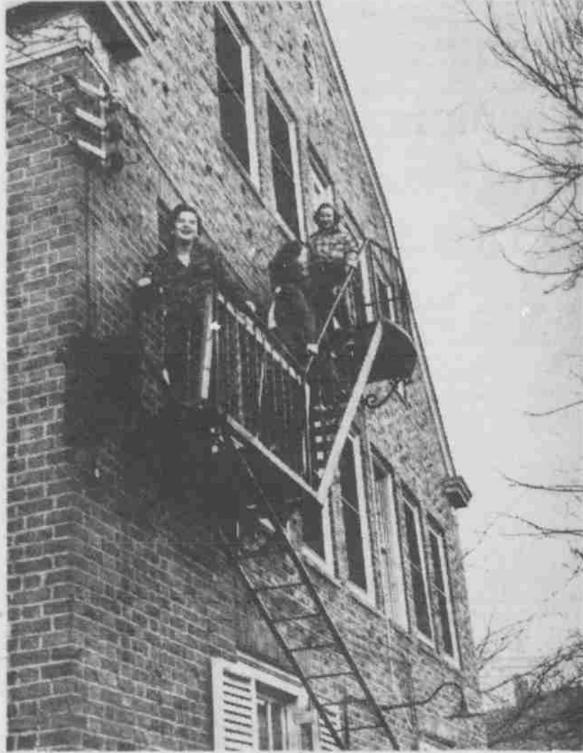
FIRE SURVEY —An experimental fire drill in one organized house revealed an astonishing ignorance of exit methods among the occupants. The four girls "escaped" from their house, via the fire escape, for the first time.
