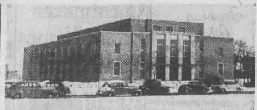
NAVAL ARMORY—One of the new university buildings to be put into use this year is the Naval Armory shown above. Located at 14th and Vine streets, this building was specially designed to harmonize with the architecture of the coliseum next to it.
