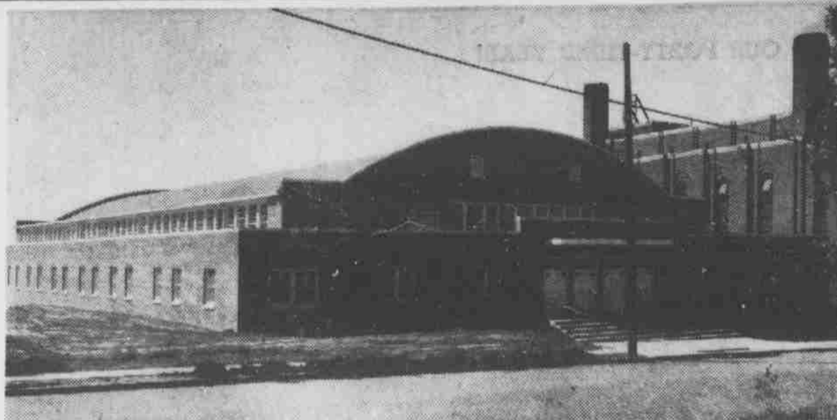
NEW INTRAMURAL HOME —Completed this summer was the new home of Intramural sports and the physical education department. Formerly an army gym at Camp Crowder, Mo., the building was secured by the University and was refaced and is ready for action.
