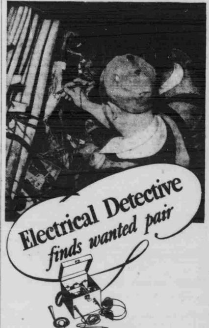
Telephone men know this piece of apparatus as the 108-A Amplifier. It is an "exploring amplifier," developed by Bell System engineers to identify pairs of wires in telephone cables-some of which contain as many as 4242 wires.
