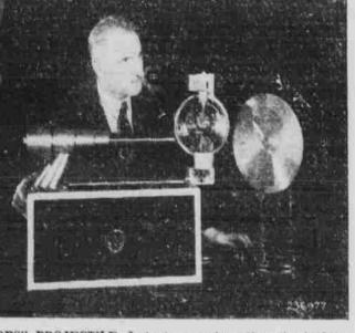
"STOPS" PROJECTILE-Instantaneous in action, the ignitron tube flashes the moment a projectile passes in front of it, thus making it possible to see action ordinarily too swift for human eyes. The devices in the picture are a compressed air gun, the ignitron tube and a target used by Dr. Phillips Thomas, Westing-house research engineer, in his locture-demonstration "ADVEN-TURES IN ELECTRICITY," that shows recent important developments of electrical engineering laboratories
