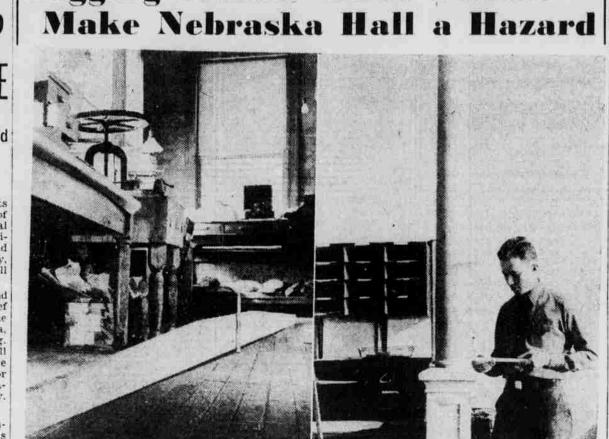
These two photographs, taken in floor in the department of conser- of one of the supporting pillars in Nebraska hall, offer mathematical vation and survey offices. The sag the military science offices. From a six foot height, the plumb line-tion of the building. In the left pic- 1 1-4 inches. In the right picture, Sergeant shows that the post leans out 1 3-4
