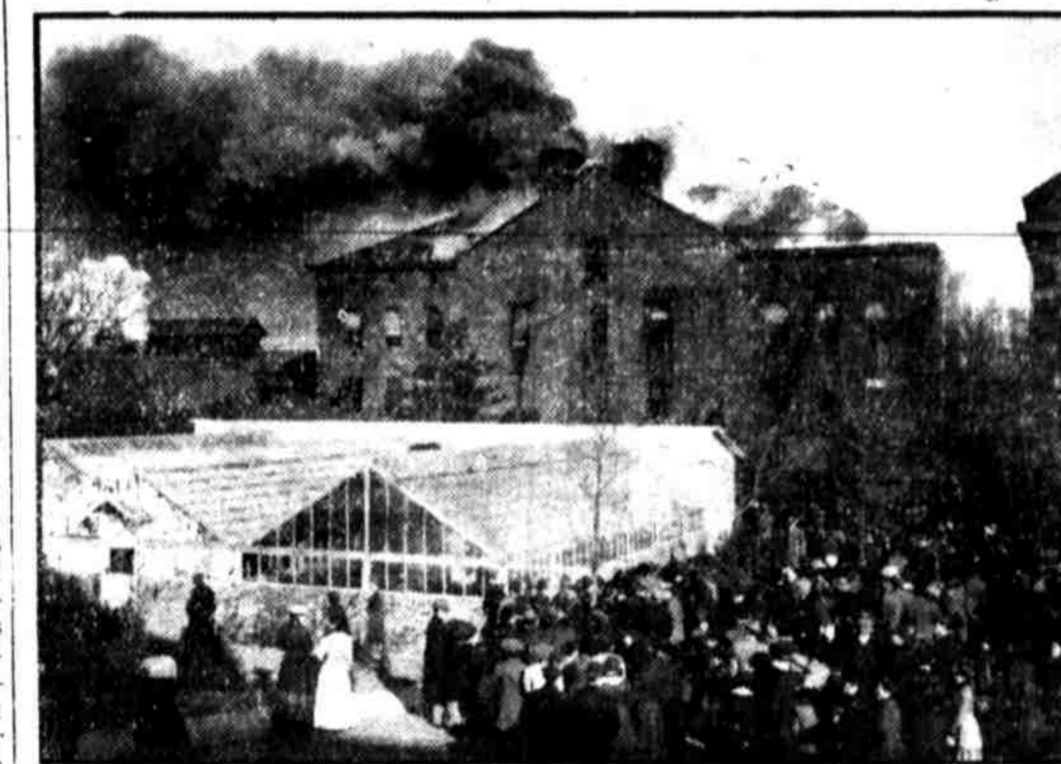
SHORTLY AFTER THE FIRE STARTED
