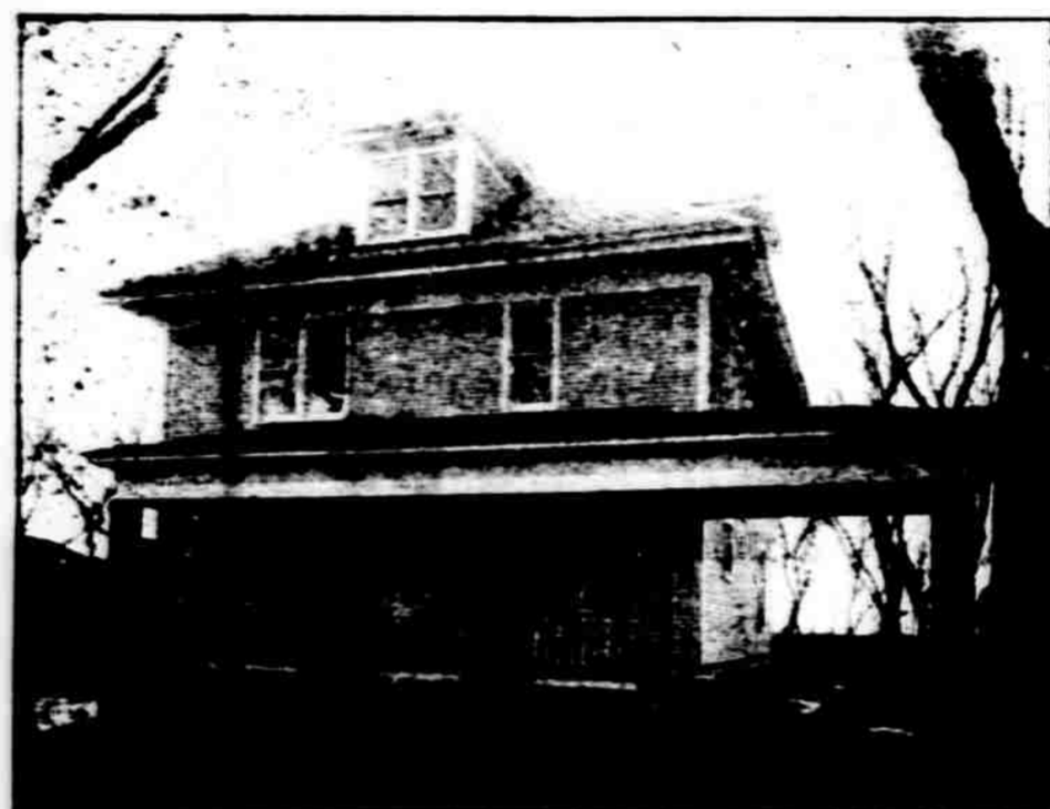
Residence of J. N. Heater nearly completed, western manager for the S. Howe Co.
