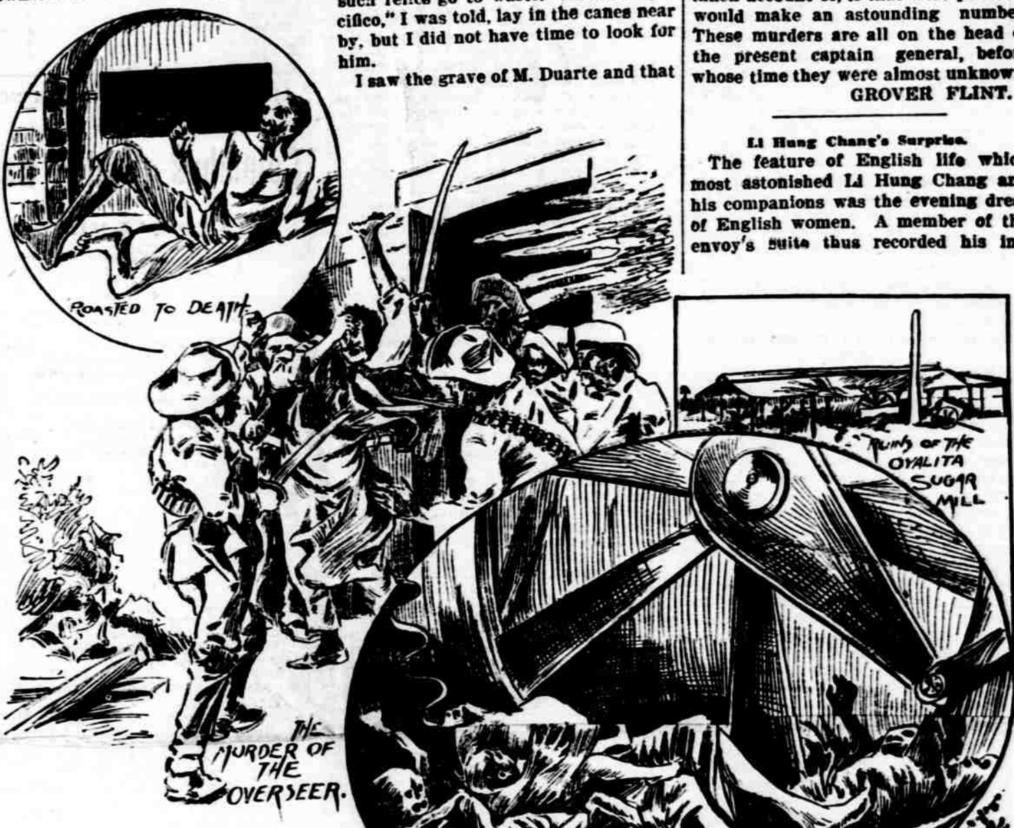
CHARRED REMAINS UNDER THE DRIVING WHEEL.
