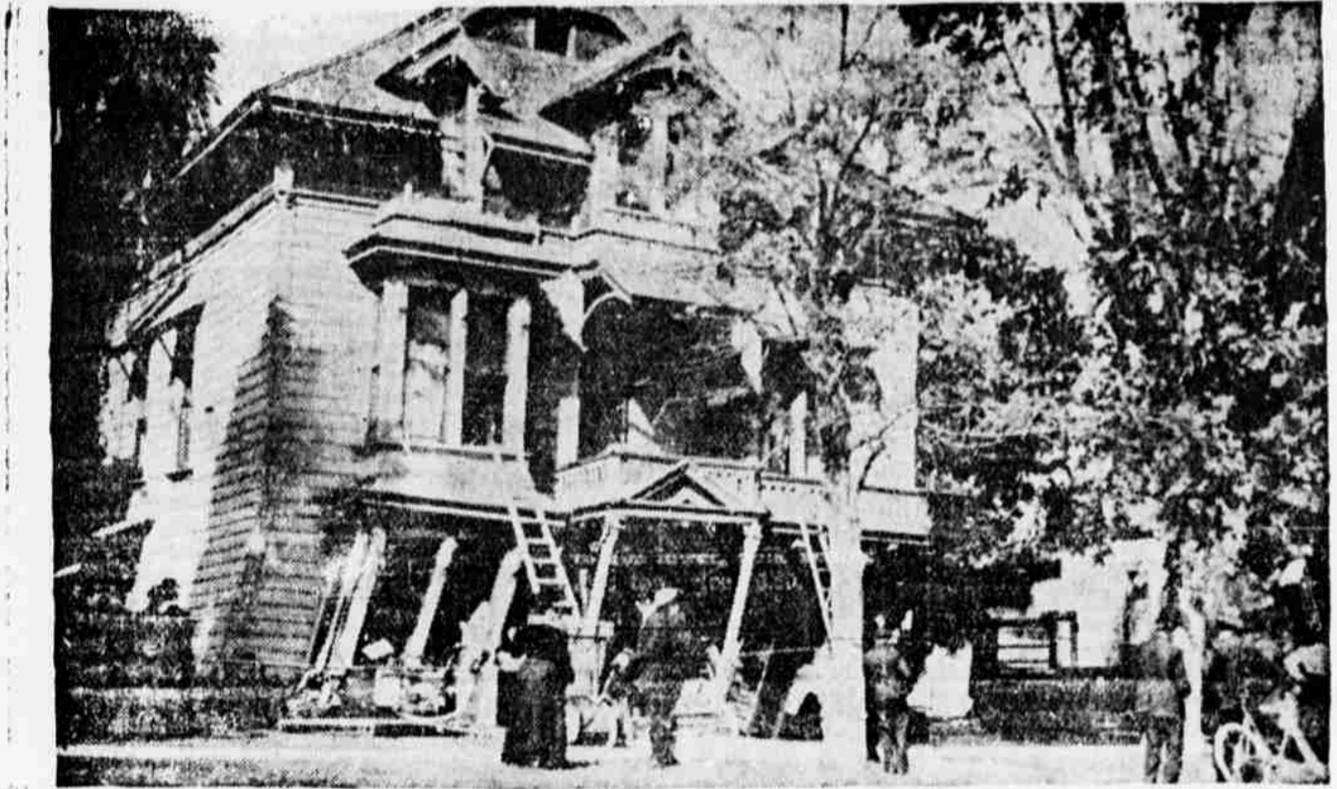
FRAME LODGING HOUSE CRUSHED BY EARTHQUAKE.
