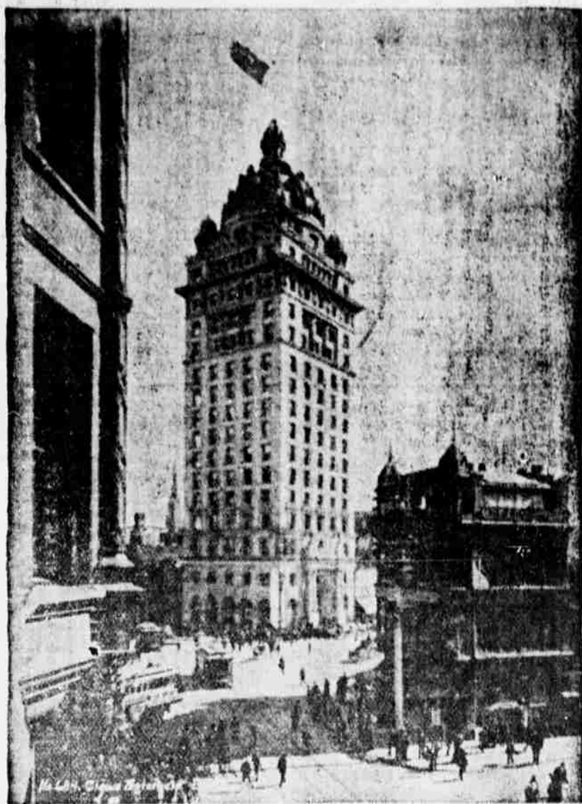
THE CALL BUILDING, ALSO DESTROYED.
